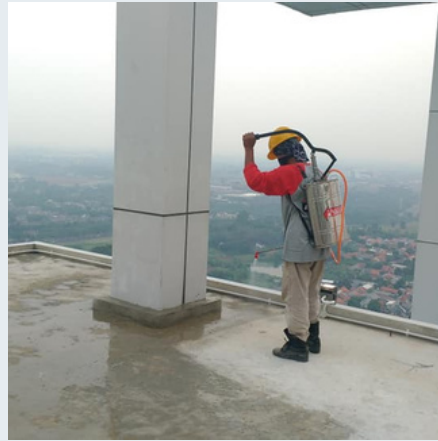
Injeksi kebocoran atap PT. Jotun Indonesia 2019
