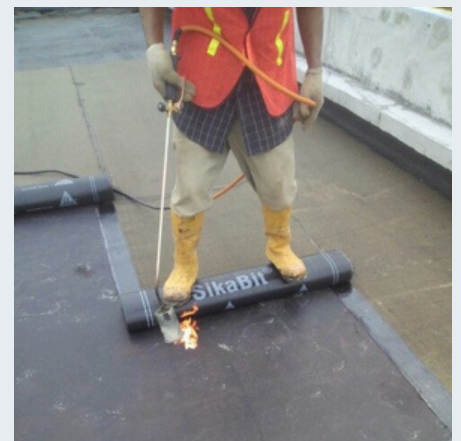
Waterproofing membrane Honda Cikampek 2021
