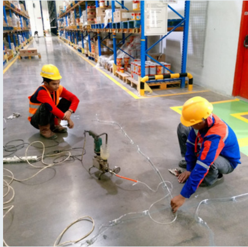
Injeksi kebocoran lantai PT. JOTUN INDONESIA
