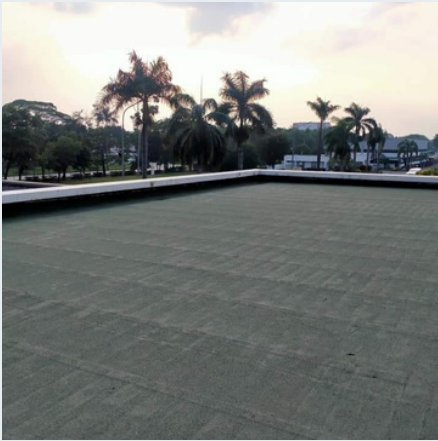
Waterproofing membrane Komp. Mesjid marakes, Ciwastra Bandung 2023
