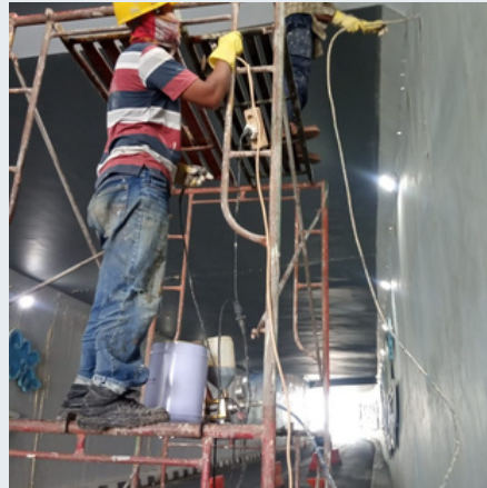
Coating gambar cat waterproofing Underpass Kota Cimahi 2021
